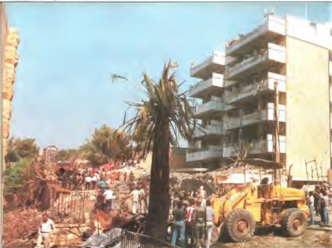
Moments after the explosion, rescue workers, American officials and Lebanese employees of the U.S. embassy cluster around the heavily damaged
